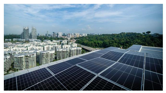
Photovoltaic panels installed on the roofs of Keppel Bay Tower and its six-storey podium block generate an energy yield of about 100,000 kWh per annum to power the building.
